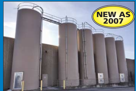
(6) 12' x 36' Imperial Industries / Novatec Model 4535 Welded Steel Silos
