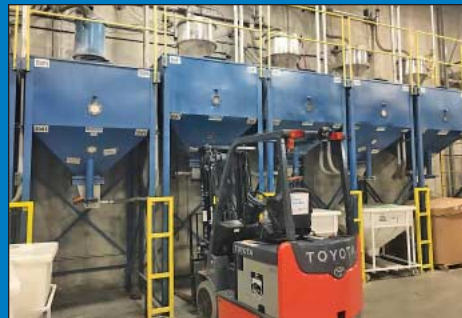
(9) 60" x 60" x 32" Novatec Cone Bottom Surge Bins
